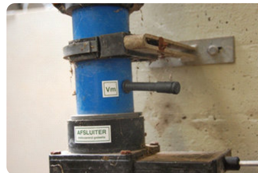
Close-up of Vm (exavct test point may vary due to local legislation)
